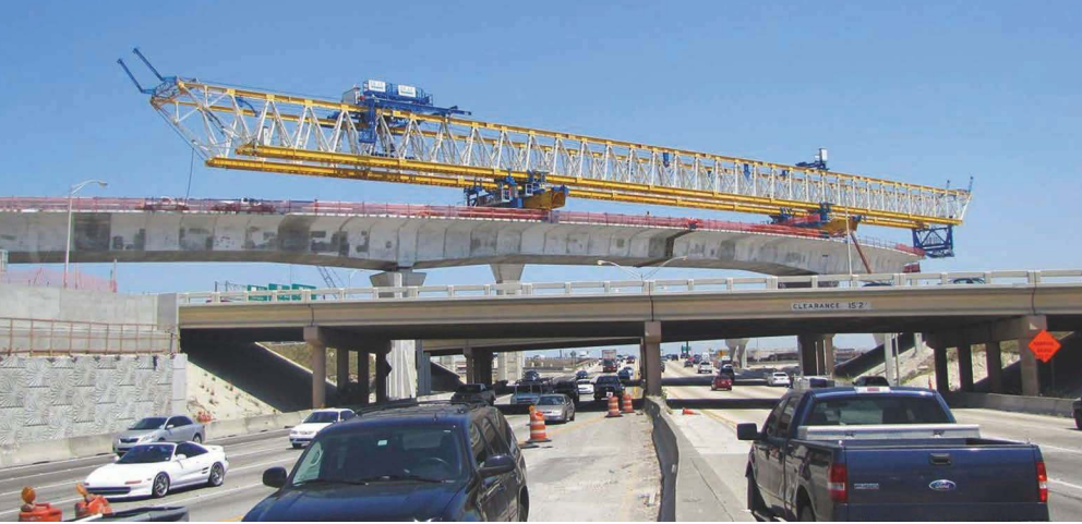
The 460-ft-long, 475-ton gantry used on the Palmetto Interchange. Photo: Condotte.
