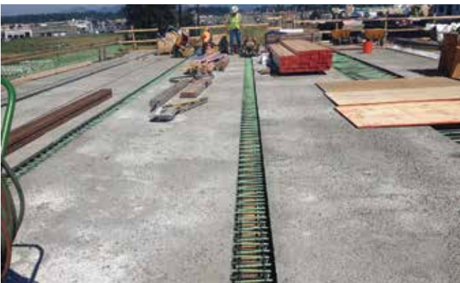
Deck closure reinforcement. Photo: Washington State Department of Transportation.
