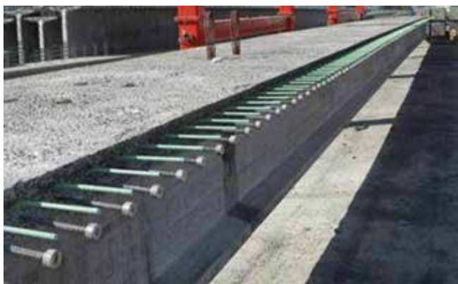
Lightweight deck bulb-tee girders in the casting yard. Photo: Washington State Department of Transportation.
