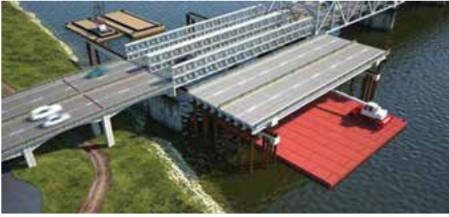
Location of replacement span during construction. Rendering: Parsons Brinckerhoff.
