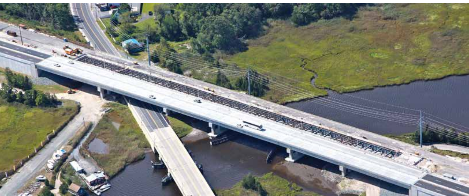
Aerial view of the Bass River Bridge. Photo: Hardesty & Hanover.
