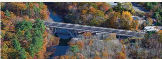
Aerial view of Stillwater Viaduct Bridge. Photo: Mark Flannary Photography.
