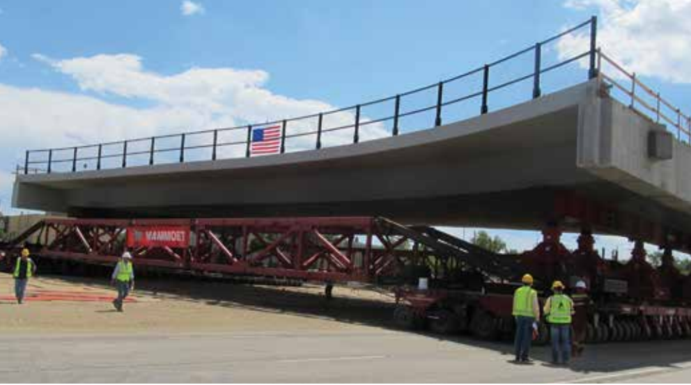
The edge of the deck and exterior webs are curved to accommodate the roundabouts at each end. Photo: Colorado Department of Transportation.
