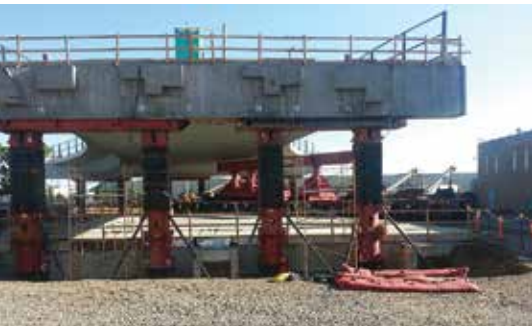
Climbing jacks at final height above ground. Photo: Wilson & Company.
