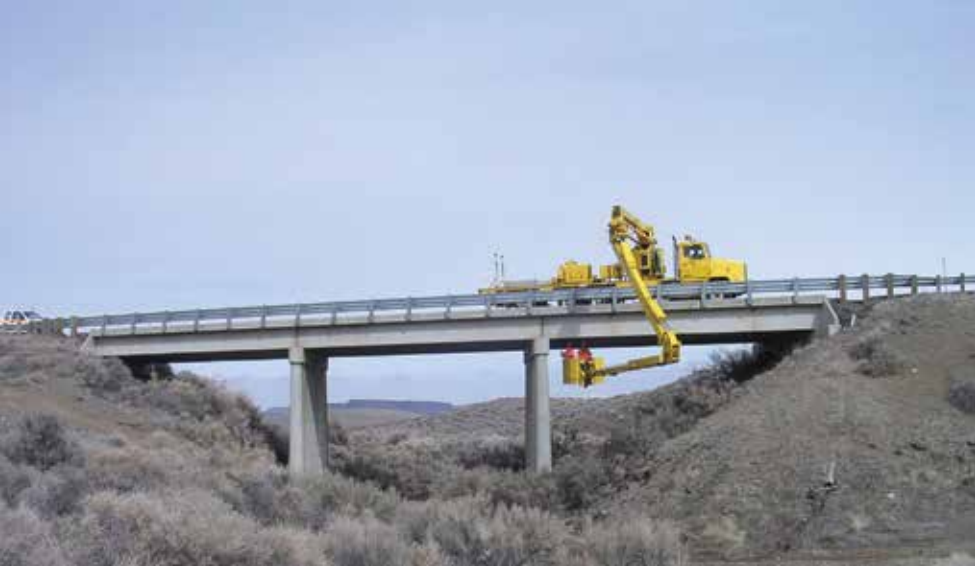
An under-bridge inspection truck is used at the site of State Highway 78 over Rabbit Creek in southwest Idaho.
