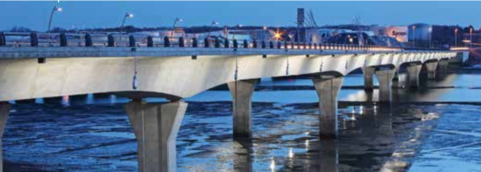
The 1610-ft-long Veterans Memorial Bridge, at a cost of $44.2 million, is the largest design-build project completed in Maine. Photo: Kimberly Brooks, T.Y. Lin.
