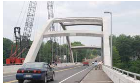
The new design of the Norridgewock Bridge consists of a three-span bridge with a cast-in-place, tied-arch center span and precast, prestressed concrete bulb-tee beam approach spans. Photo: Maine Department of Transportation.
