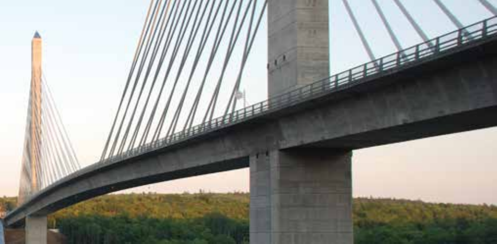
The Penobscot Narrows Bridge in Waldo and Hancock Counties, a cast-in-place concrete segmental cable-stayed bridge, was created when renovation plans showed needed repairs were too extensive. The distinctive bridge was completed in just 30 months. Photo: Maine Department of Transportation.
