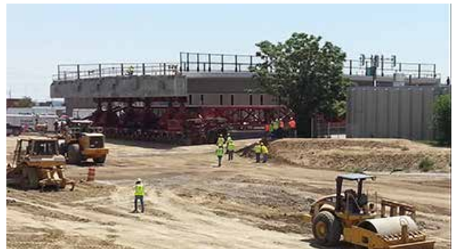
The edge of the deck and exterior webs are curved to accommodate the roundabouts at each end.
