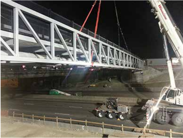
Pedestrian bridge placement over I-70. Photo: Wilson & Company.
