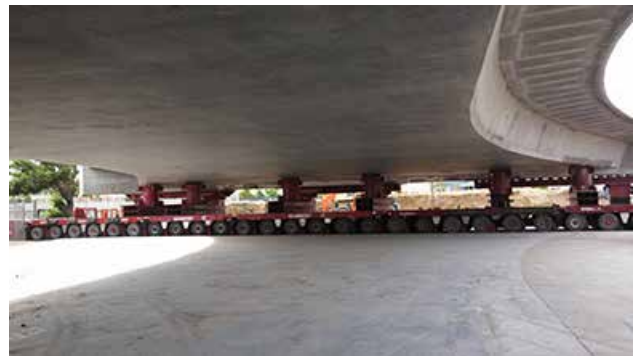
The edge of the deck and exterior webs are curved to accommodate the roundabouts at each end.
