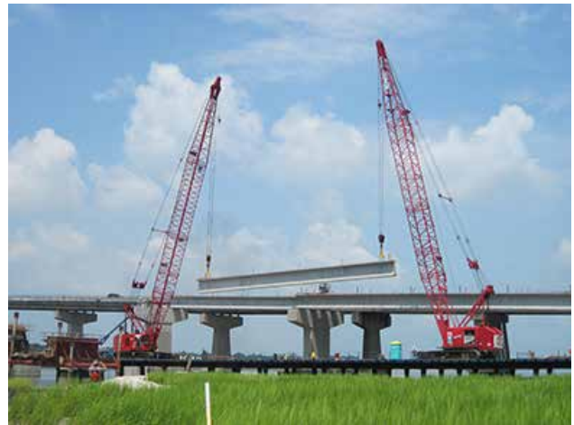
Record-setting 96-in.-deep main-span, bulb-tee beams being set. Photo: United Contractors.
