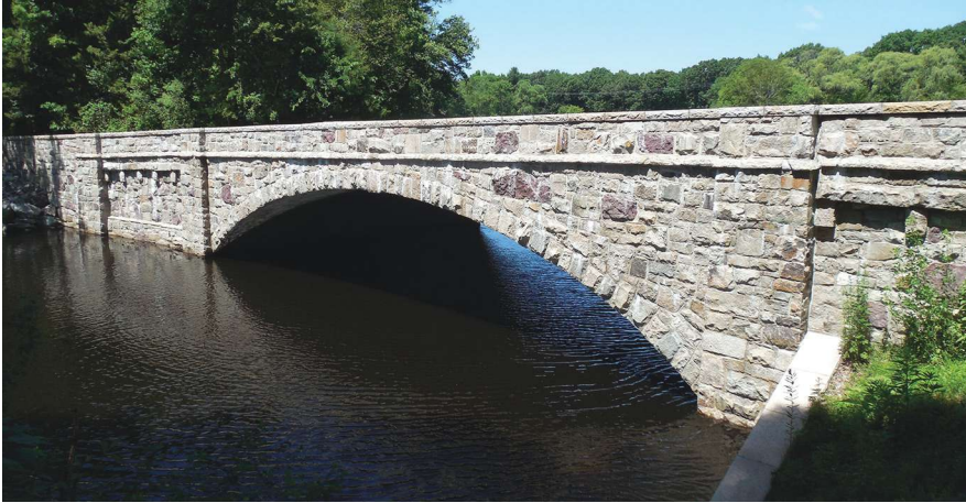
The completed Willow Street Bridge. Photo: John Phelan.
