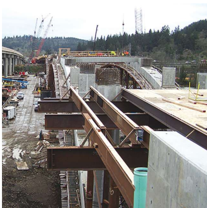
Approach span falsework and formwork plus bent 2 column reinforcement.
