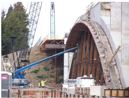
Arch and approach span falsework for the I-5 Whilamut Crossing Bridges.
