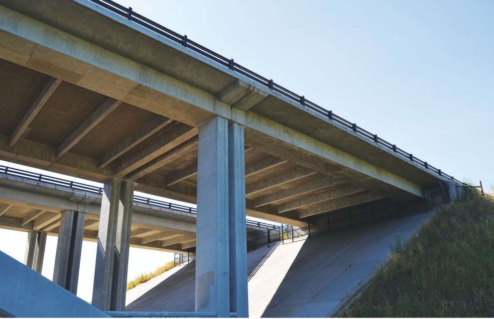
View of the north approach span.
