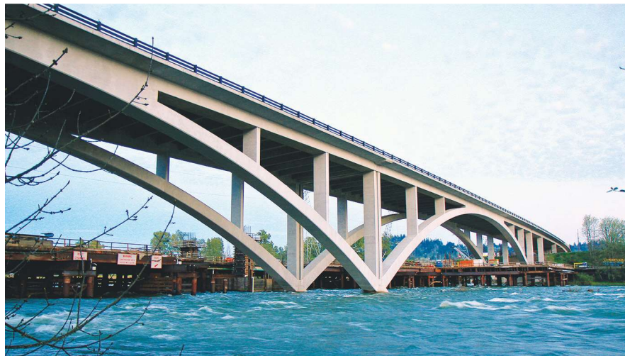
Completed southbound I-5 Whilamut Crossing Bridge looking toward south approach spans, with northbound work bridge in the background.
