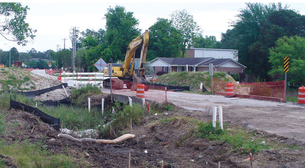
Old Bowman Road Bridge prior to demolition.
