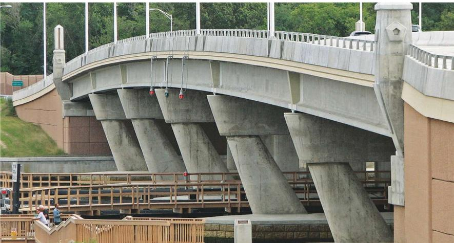
as possible to simplify the architectural concept and minimize the duration of in-water construction. The bridge was built with precast concrete pier cofferdams, columns, cap beams, and bulb-tee girders. (For more on this project, see the Fall 2009 issue of *ASPIRE*.™)
