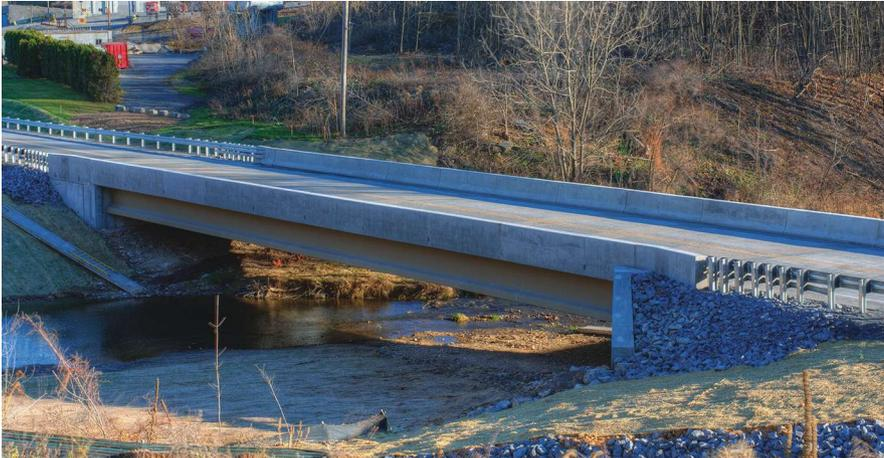
The Ashcom Cove Creek Bridge in Bedford County, Pa., consists of five 120-ft-long precast concrete bulb-tee girders and a total-precast concrete structure. Photo: PennStress.
