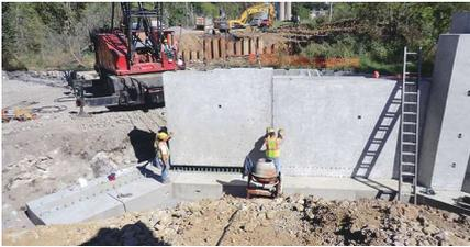
Workers place precast concrete abutments for the Ashcom Cove Creek Bridge. Photo: PennStress.
