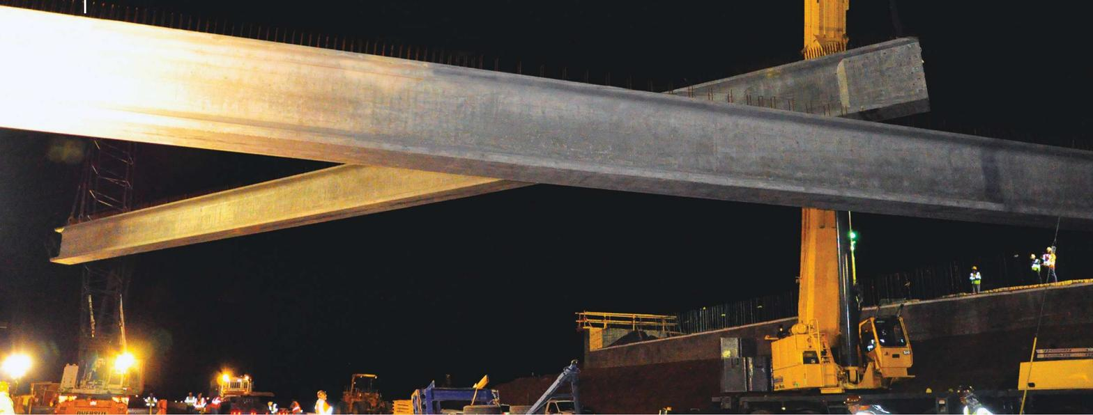
Positioning of the second wide-flange precast concrete girder for placement at the Riego Road Overcrossing. Photo: Brandi Matteoni.
