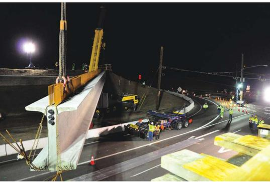
Setting the first of 14 California wide-flanged girders into the second span. Extensive shear reinforcement is required for the girder-slab connection adjacent to the bent cap so that the integral bent cap behaves as desired during a seismic event. Photo: Brandi Matteoni.
