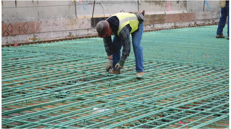
Placing of epoxy-coated reinforcing steel. Photo: Epoxy Interest Group of CRSI.
