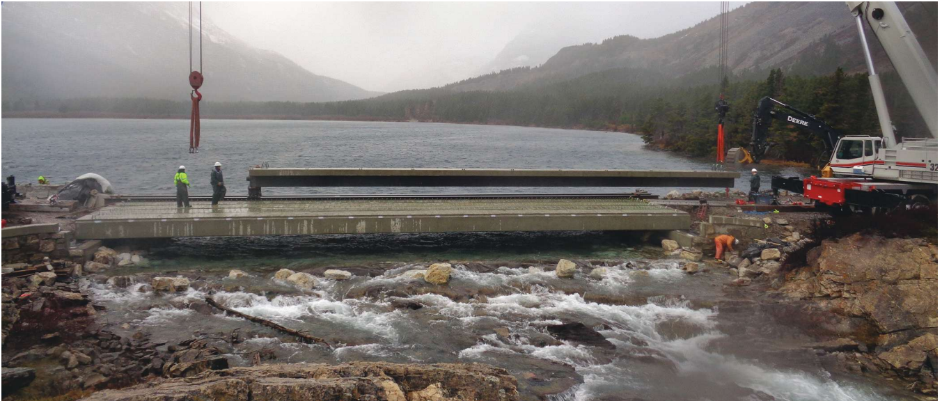
New bridge being installed. Photo: Sam Barchus, Northbank Civil & Marine.
