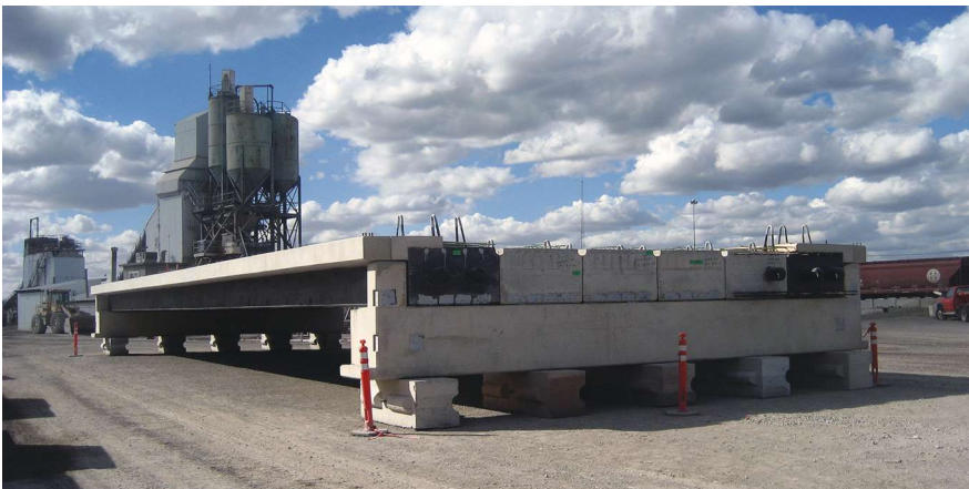
Trial fit in precast yard. Photo: Linda Josephson, Oldcastle Precast Inc.
