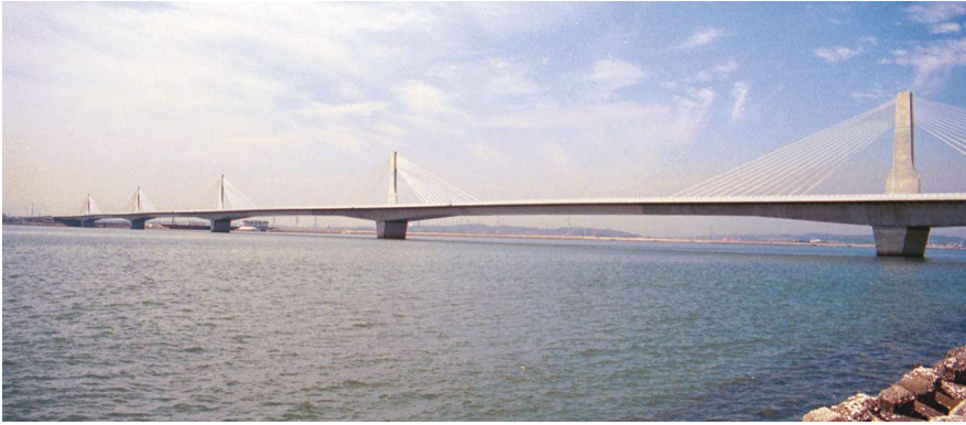
Ibi River Bridge, Japan, is a multi-span, extradosed prestressed concrete bridge. Photo: Steven Stroh.
