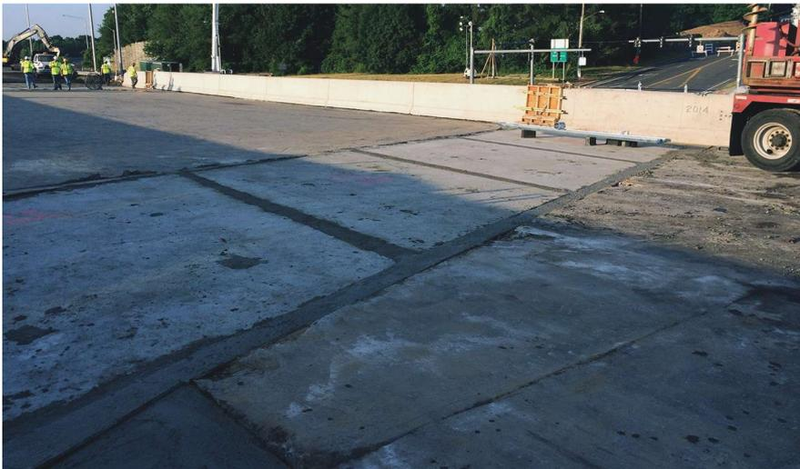
Precast concrete approach slabs, cast-in-place concrete deck, and parapet closure placements being prepared for final paving for the I-84 Bridges over Marion Avenue.
