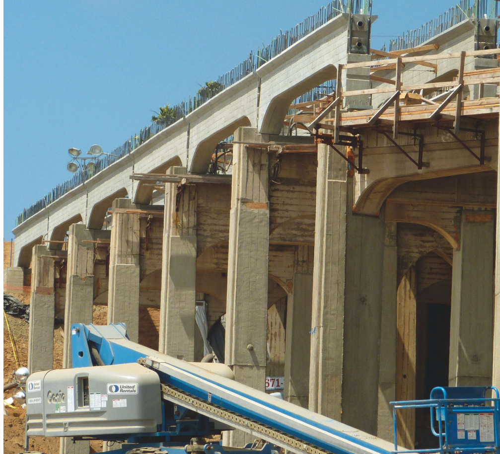
Precast concrete girders erected on rehabilitated substructure.
