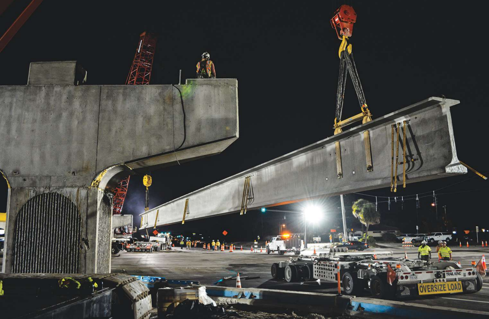
Lifting of a 209-ft-long Florida I-beam. Photo: Lane Construction.
