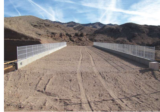
A wildlife fence channels sheep toward the overpass. Photo: Arizona Department of Transportation.
