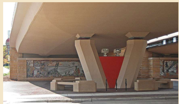
Figure 2. Daylight and space at the south abutment. Photo: Frederick Gottemoeller.
