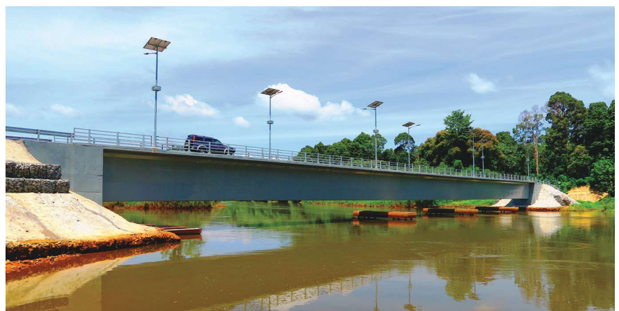
Figure 4. Batu 6 segmental box-girder bridge with 100 m (328 ft) span.
