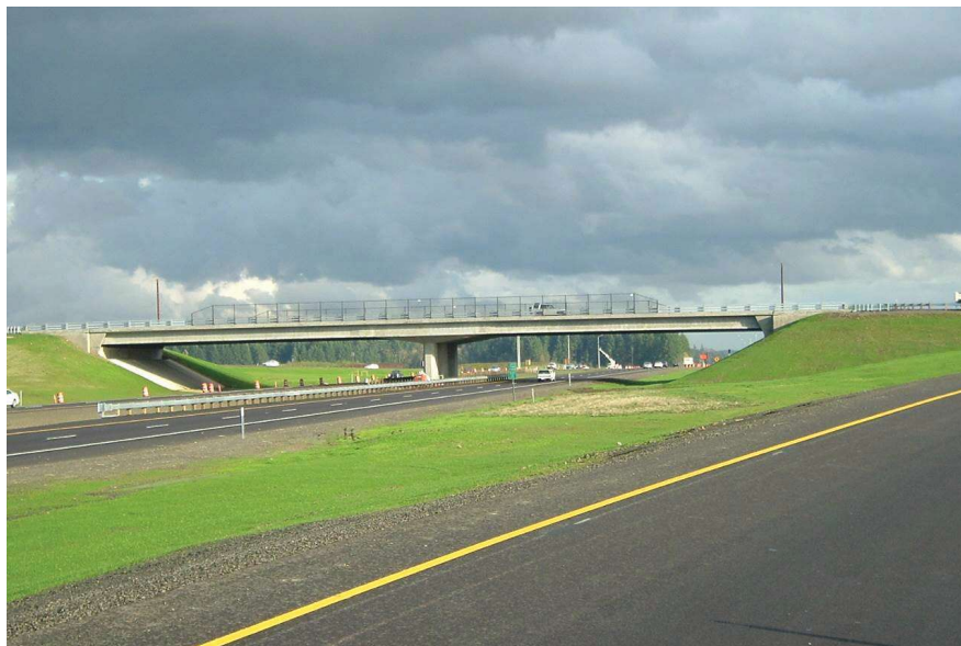
Jackson School Road over Highway 47 Bridge used for comparison of Grade 60 and Grade 80 reinforcement for the reinforced concrete deck.
