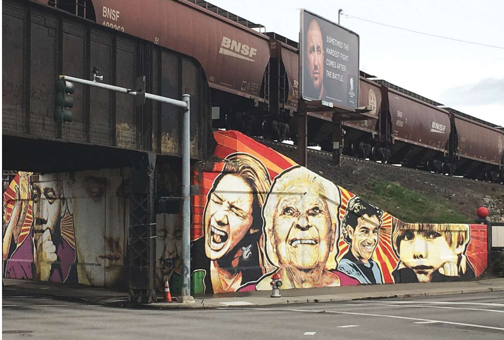
Railroad bridge in Spokane, Wash., demonstrating territorial reinforcement and tendency of taggers to respect public art. Photo: Washington State Department of Transportation.
