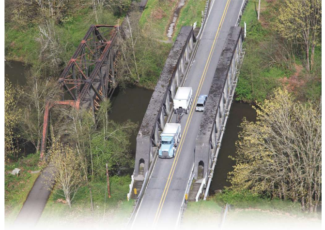
State Route 162/6 existing historical concrete pony truss bridge that was replaced. Photo: Washington State Department of Transportation.
