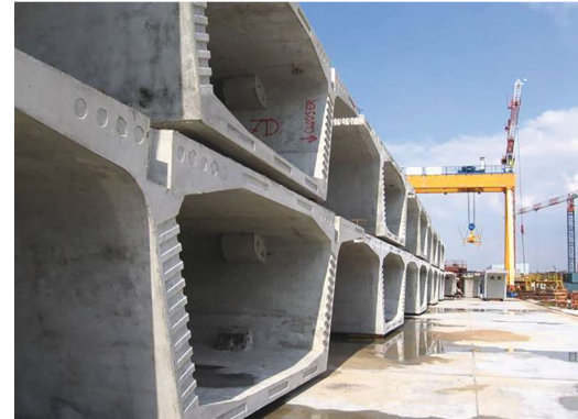
Casting yard. Photo: Finley Engineering Group Inc.
