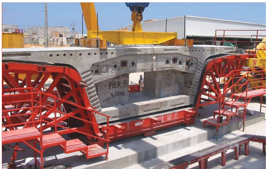
Precasting machine. Photo: Finley Engineering Group Inc.
