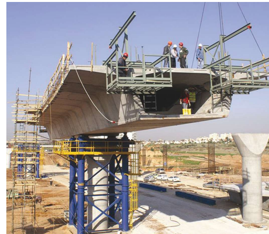
Segment erection. Photo: Danya Cebus.
