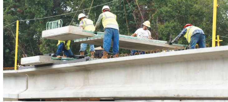
Precast concrete overhang panel placement.
