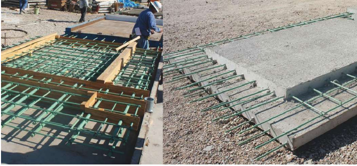
Precast concrete overhang panel fabrication and completed panel.
