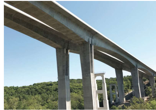
Jeremiah Morrow Bridge, with cast-in-place concrete segmental box girders, is the tallest bridge in Ohio. All Photos: Ohio Department of Transportation
