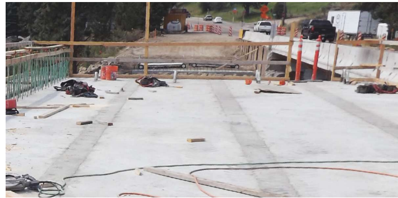
Deck surface after girder closure pours have been completed.
