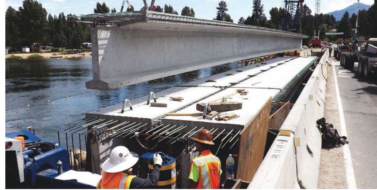
Stage 1 deck girder erection from existing bridge.
