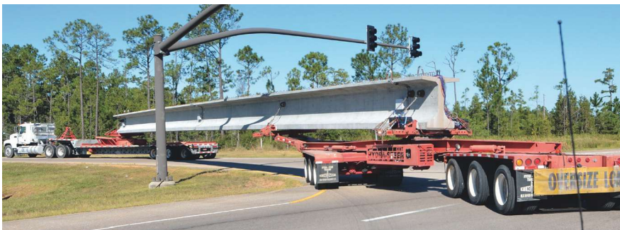
Girder turning onto an interstate ramp, an example of a significant event causing differential bending strain at the top flange of the girder.
