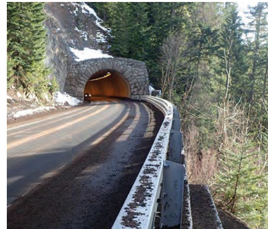
This photo shows westbound traffic exiting the west tunnel portal. A completed half viaduct carries east bound traffic into the tunnel. Photo: ODOT Region 2.
