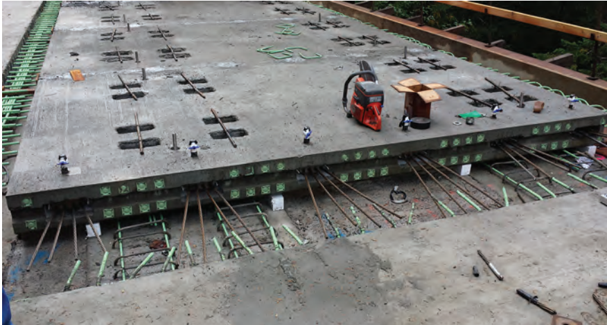
Precast concrete deck panel with joint and pocket details visible. Photo: Knife River Corporation.
