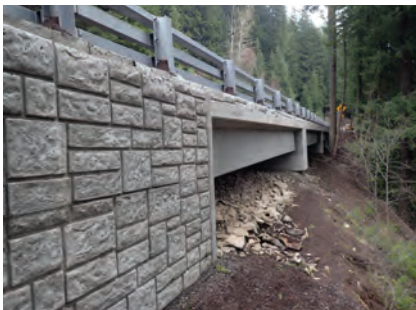
Typical elevation of completed half-viaduct bridge. Photo: ODOT Region 2.
