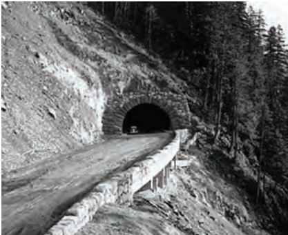
A 1933 construction photo at the Salt Creek Tunnel's west entrance with a half-viaduct bridge visible. Photo: Oregon State Archives.
