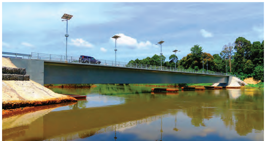
Batu 6 segmental box-girder bridge with 100 m (328 ft) span. Photo: DURA Technology.
