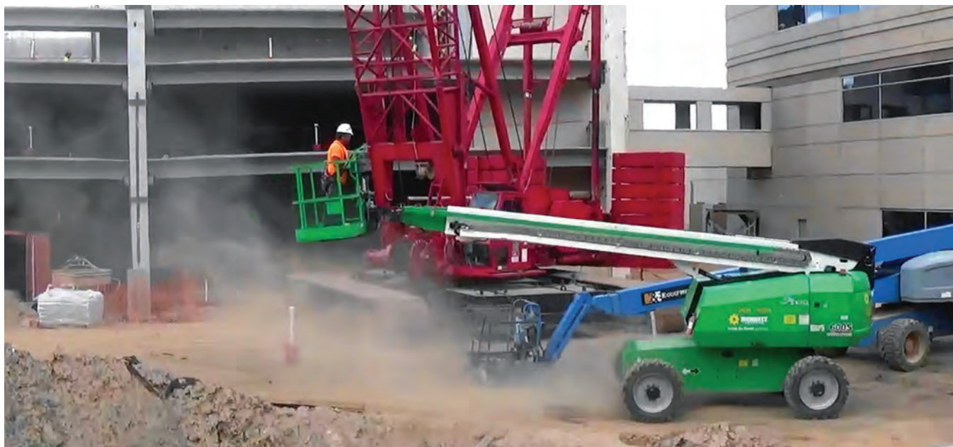
An equipment operator works in a common jobsite area.
