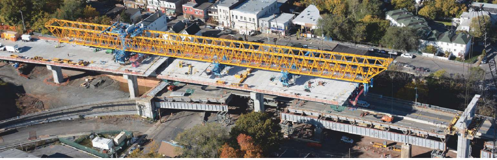
Balanced-cantilever construction for the Bayonne Bridge approaches.
