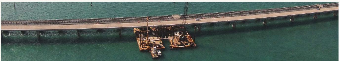
Aerial view of the barges in position for V-pier installation. All Photos: James Charles.
