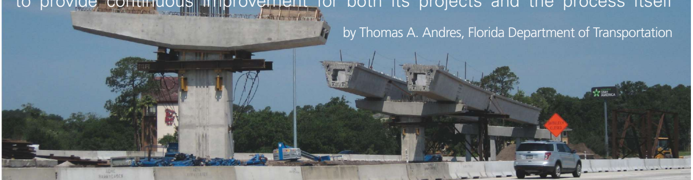
Florida Department of Transportation's J. Turner Boulevard/Interstate 95 design-build project features a curved, spliced U-girder structure. Photo: Florida Department of Transportation.
