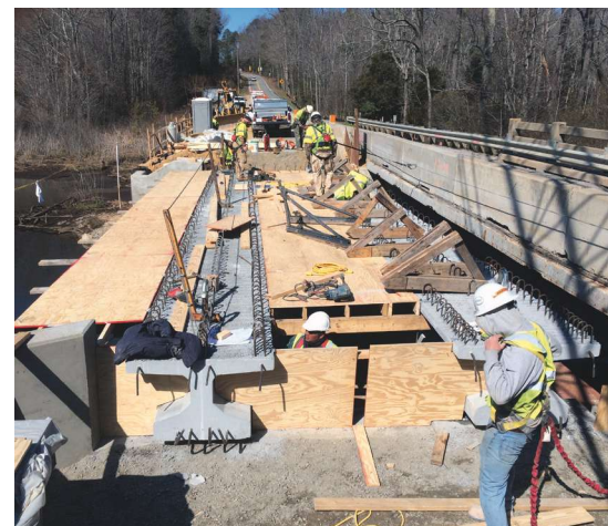
Two 29-in.-deep lightweight concrete bulb tees prior to deck placement. Photo: Virginia Department of Transportation.
