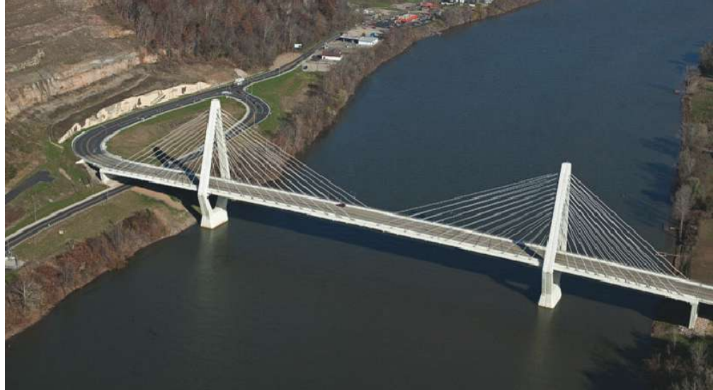
The Bridge of Honor over the Ohio River is a cast-in-place segmental concrete cable-stayed bridge designed and built by the Ohio Department of Transportation and then turned over to the West Virginia Department of Transportation for operation and maintenance.
