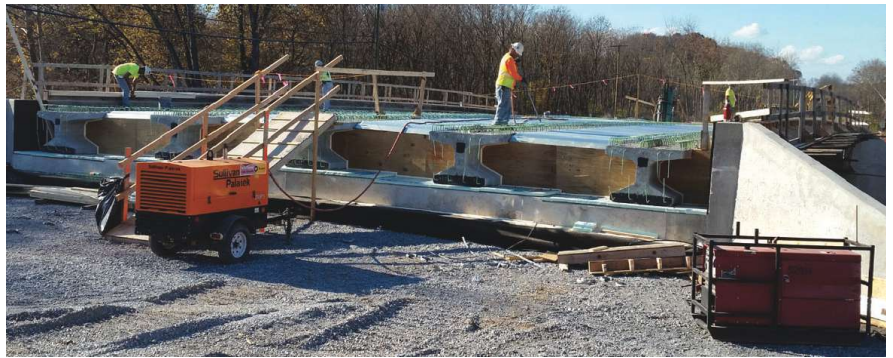
The Van Metre Ford Bridge (above and below), a design-build project, contains prestressed concrete hybrid bulb tees with a 40-in.-wide bottom flange that allows more prestressing strands to be used.
