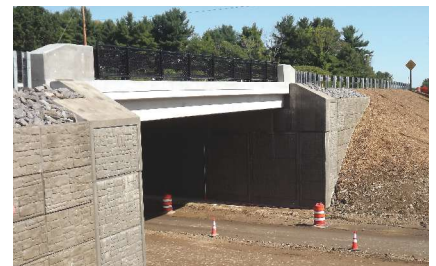
Simple span NEXT beam in Kittery, Maine.
