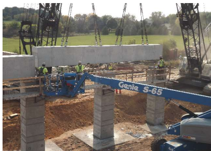
Precast concrete pier cap being placed on precast columns in Wisconsin.
