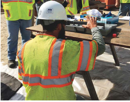
Unit weight testing of grout by mud balance.
