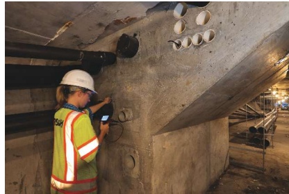
Post-grouting visual inspection using a borescope.
