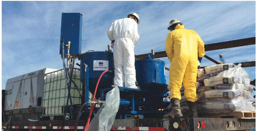
Grout mixing operations. All Photos: RS&H.
