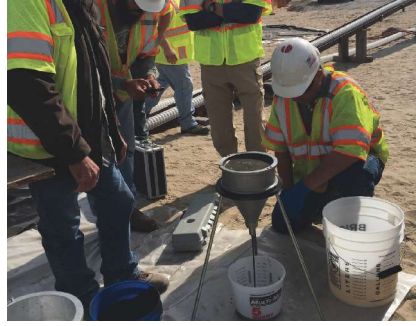
Flow cone testing of grout.
