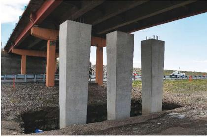
The cast-in-place concrete pier columns are complete and await demolition of the existing bridge. Photo: Fernando Quiroga.
