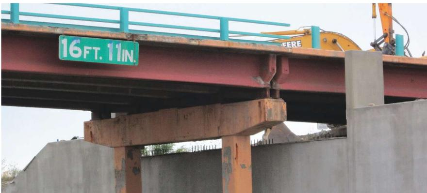
A substantial portion of construction of the cast-in-place abutment and retaining walls was completed while the existing bridge remained in service. Photo: Tom Cartner.
