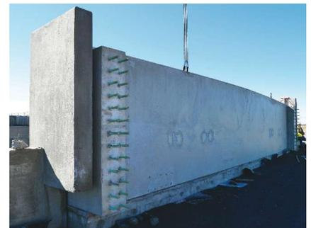
After demolition of the existing bridge, the precast concrete abutment cap with back wall is placed on the abutment wall. The bar extensions will extend into the bar splice sleeves embedded in the precast concrete wingwalls. Photo: Fernando Quiroga.
