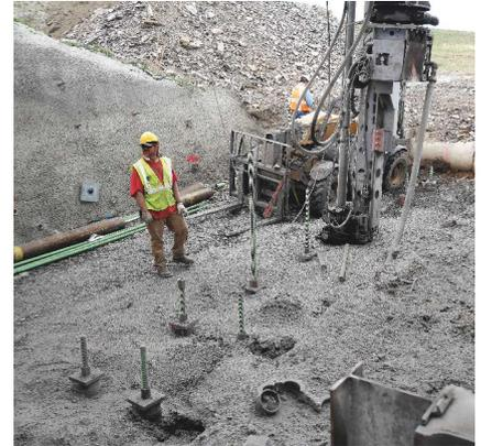
Drilling for micropiles proceeds under the shadow of the existing bridge. The single no. 14 reinforcing bar in each pile is supported on the top of the steel casing. The temporary soil-nailed retaining wall is in the background. Photo: Fernando Quiroga.
