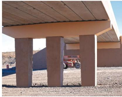
The cast-in-place concrete pier columns and precast concrete pier cap are shown in the foreground with the cast-in-place concrete retaining and abutment walls with precast concrete abutment cap in the background. Photo: Fernando Quiroga.
