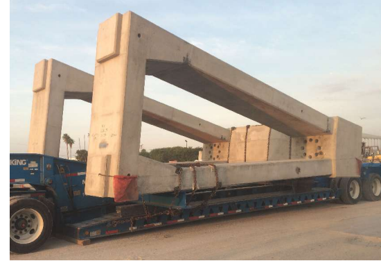
Precast concrete replacement pier ready for transportation from precaster's plant in Tampa, Fla. Photo: Kurt Podoll, Standard Concrete.
