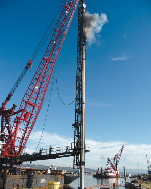
Driving 24-in.-octagonal prestressed concrete piles at Pier 4, Port of Tacoma, Wash.
