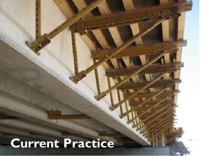
Figure 1. The current deck overhang bracket system and the proposed precast concrete overhang system.. All Figures and Photos: Sean P. Clifton.
