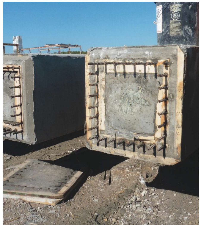
The Louisiana Department of Transportation and Development (LaDOTD) required a new corrosion-resistant detail for both ends of the piles to attain a 100-year service life. The detail required that the stainless steel strands be recessed 2 in. at each end and the recess be filled with cementitious grout.
