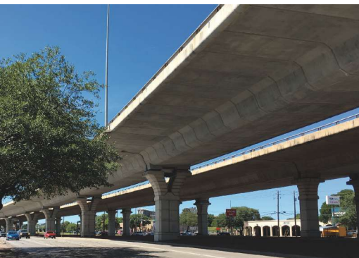
Precast segmental concrete box girder for U.S. Route 183 elevated viaduct, Austin, Tex. Photo: Oguzhan Bayrak.
