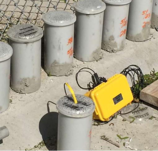
Sensors at the Black Ankle Valley Bridge were also used to monitor test cylinders for curing compliance and verification of strengths.
