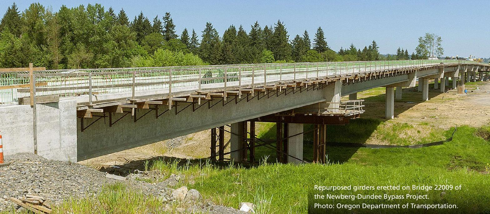
Repurposed girders erected on Bridge 22009 of the Newberg-Dundee Bypass Project.
