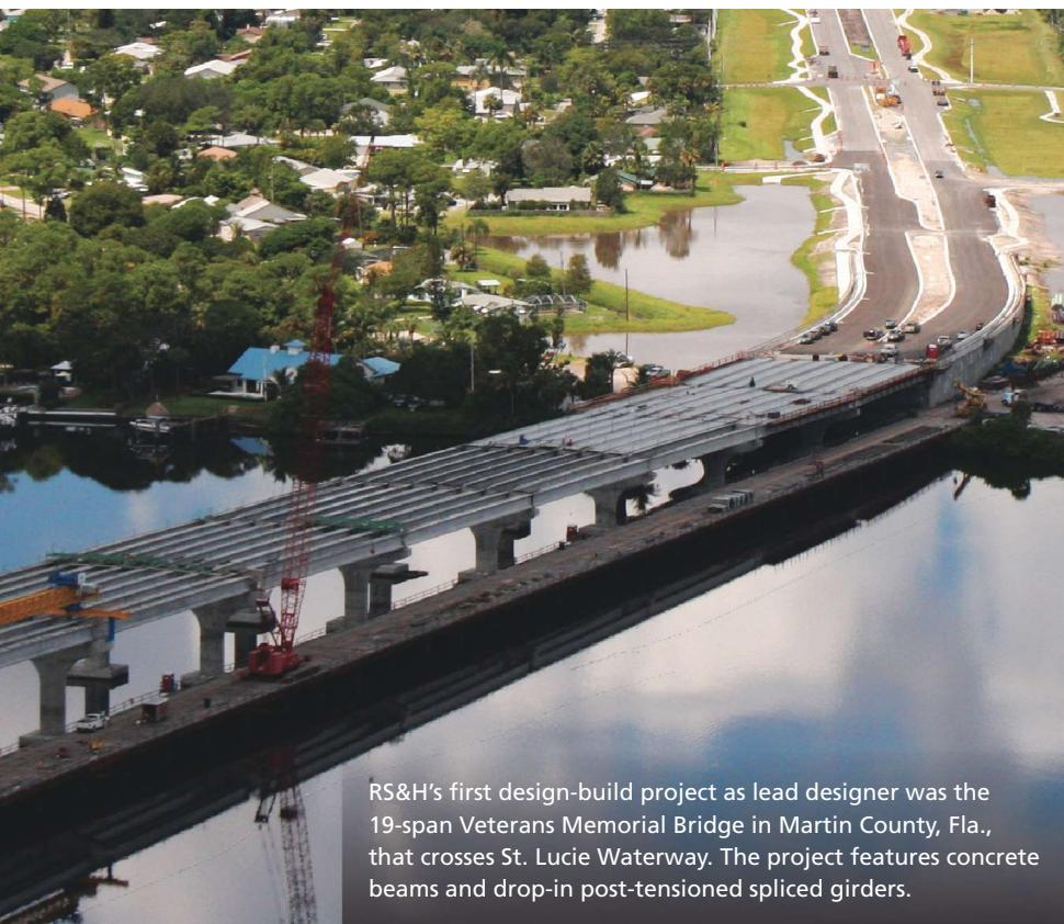
RS&H's first design-build project as lead designer was the 19-span Veterans Memorial Bridge in Martin County, Fla., that crosses St. Lucie Waterway. The project features concrete beams and drop-in post-tensioned spliced girders.
