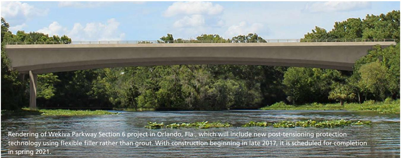
Rendering of Wekiva Parkway Section 6 project in Orlando, Fla., which will include new post-tensioning protection technology using flexible filler rather than grout. With construction beginning in late 2017, it is scheduled for completion in spring 2021.
